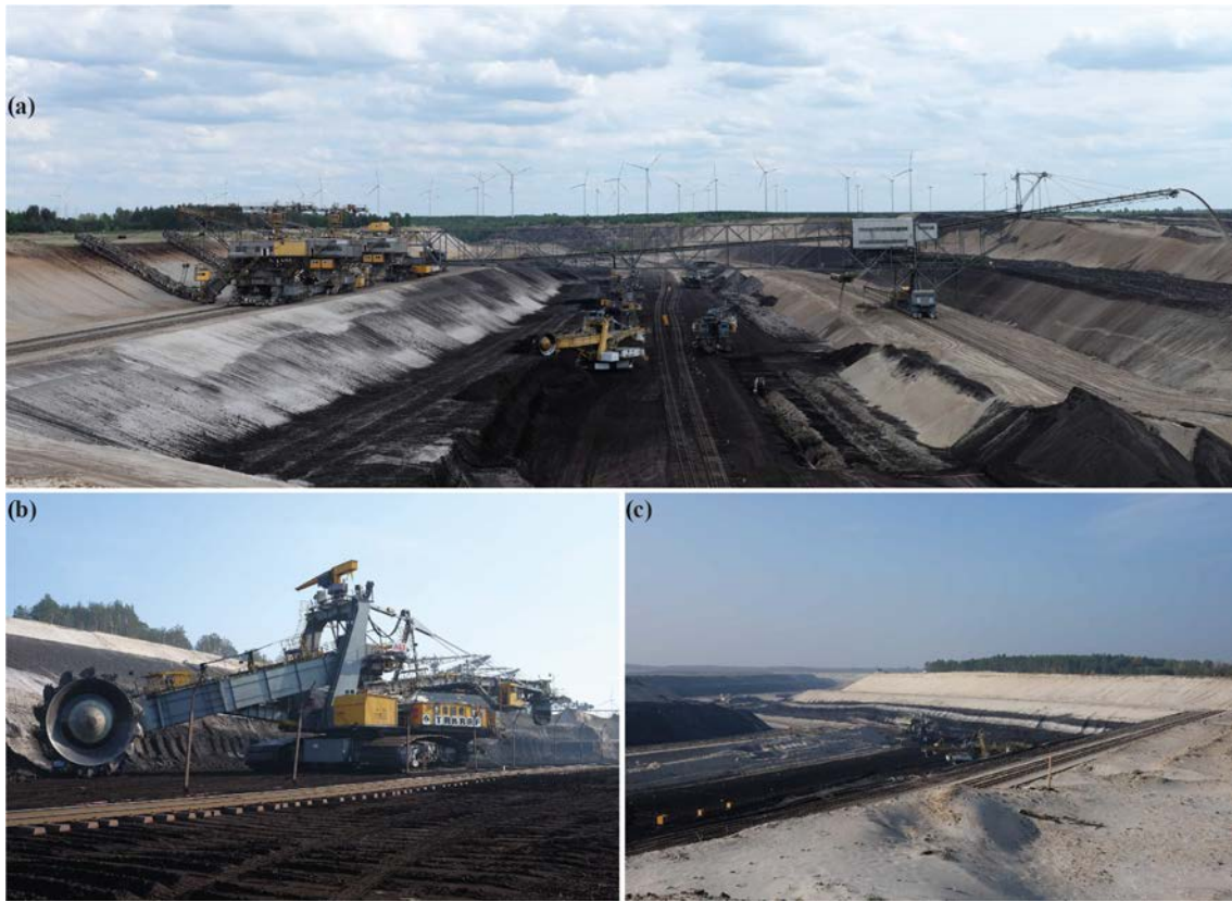
Figure 7. Conveyer bridge and excavators of the open-cast mine Cottbus-Nord.
