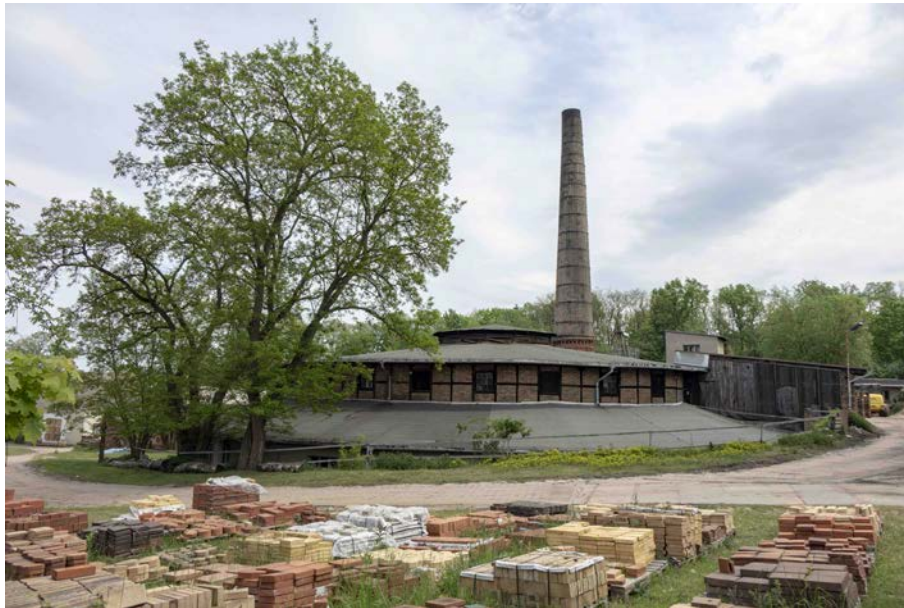
Figure 8. Ring furnace of a brick manufactory in the Glindow Alps ( 52^{\circ}21.3' \text{ N} , 12^{\circ}55.4' \text{ E} ) (photo: Bernhard Diekmann, 2020, with courtesy of the Brickyard Museum of Glindow).
