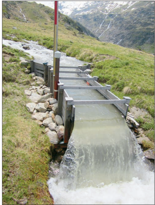
Fig. 10: Automatic gauging station at the meltwater stream of the Hochebenkar rock glacier near Gurgler Alm at an elevation of 2220 m.
